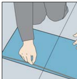
Run a chalk line across the room passing through the centre point and following the edge of the tiles.
